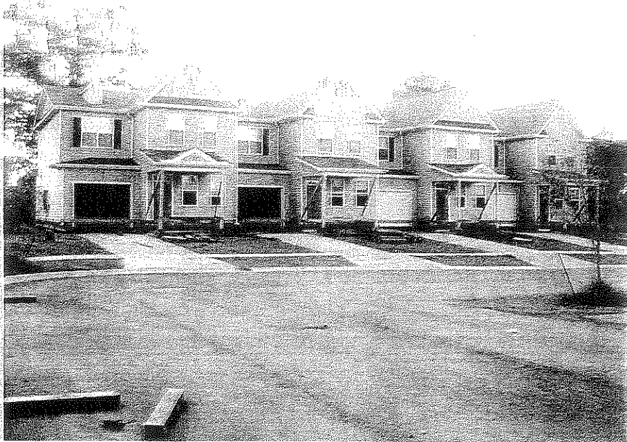
Bandolier Circle, 1357, All Support Beams Installed, 09/12/08
